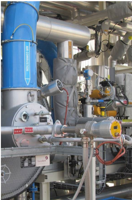
Pillard flame scanners fitted on industrial burners
